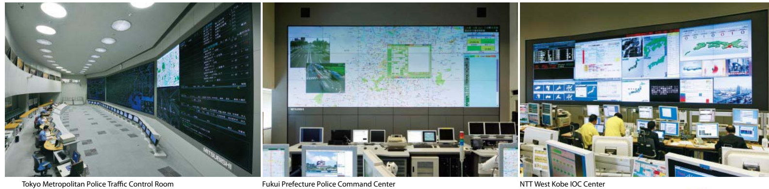
Tokyo Metropolitan Police Traffic Control Room
